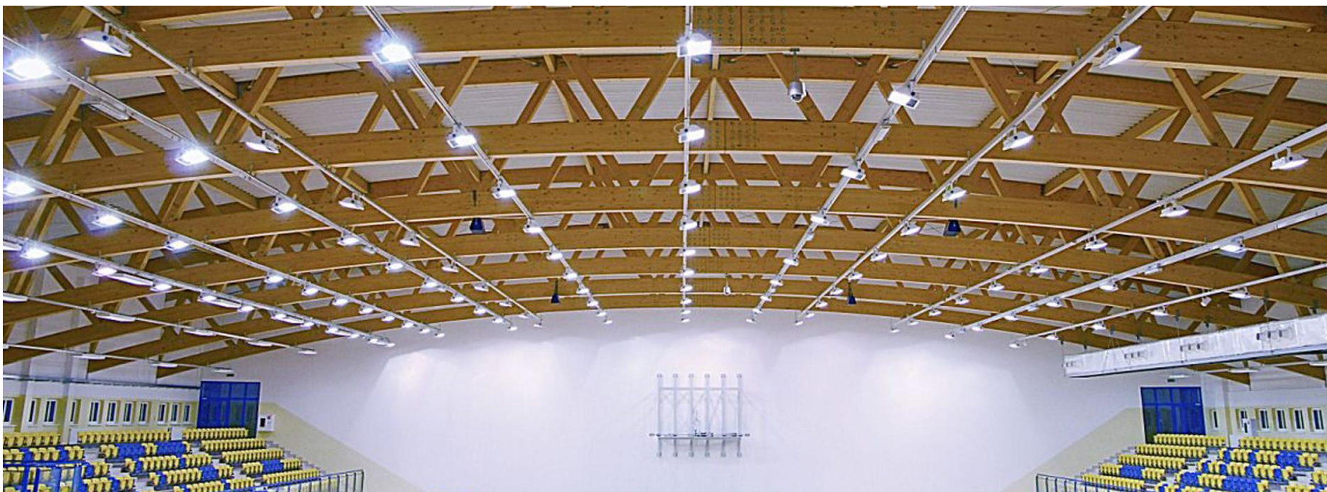
KATTOWICE SPORTS HALL POLAND
